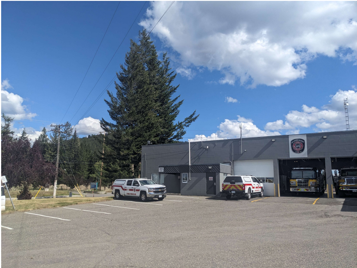
Figure 3: The 100 Mile House Fire Hall
