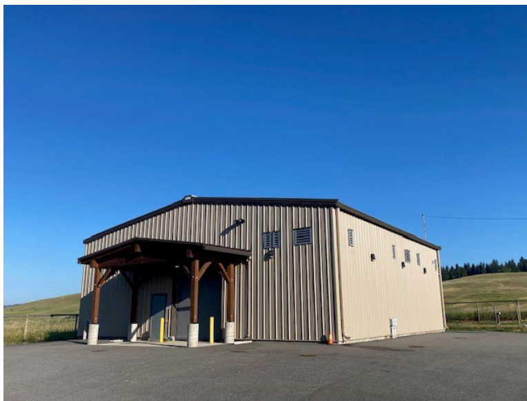
Figure 1: The District of 100 Mile House Water Treatment Plant
