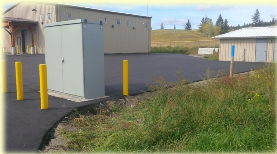
Well #4 Upgrade - Water Treatment Plant
