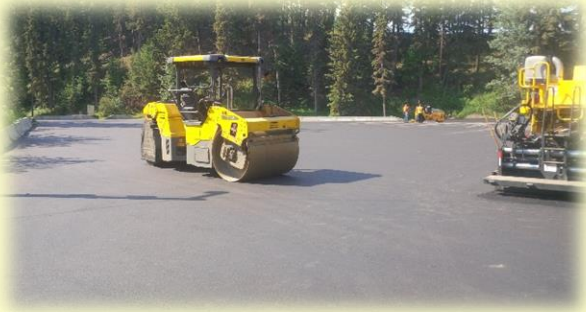
Parking Lot Paving
