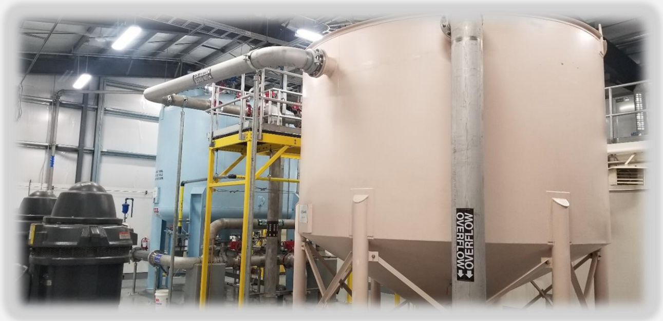
A Look Inside the Water Treatment Plant
