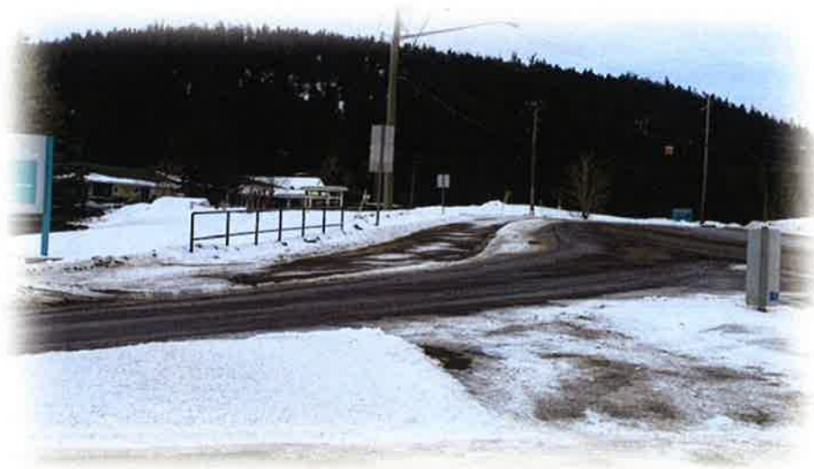
A Winter Look at the new sidewalk on Horse Lake Road from Cedar Avenue to the Bridge
