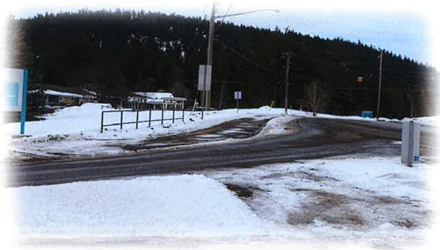
A Winter Look at the new sidewalk on Horse Lake Road from Cedar Avenue to the Bridge
