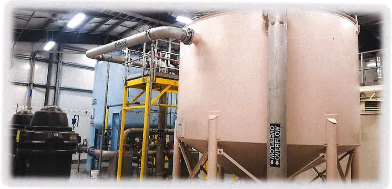
A Look Inside the Water Treatment Plant
