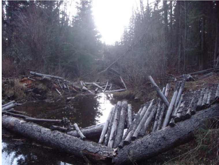
Figure 6 – Old Scott Creek Bridge
