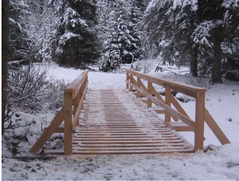
Figure 7 - Scott Creek Bridge
