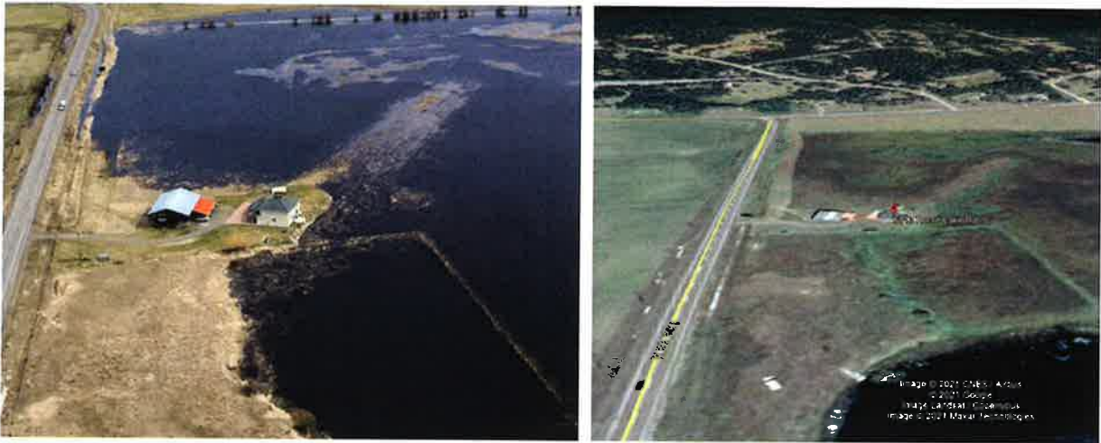
Figure 1-2. Flood inundation at 6013 Horse Lake Road near the outlet of Bridge Creek into Horse Lake, looking North (within the CRD). The Google Earth Image shows the banks of Bridge Creek at the same location, for comparison. (May 2, 2020, Photo Courtesy CRD, 2020).
