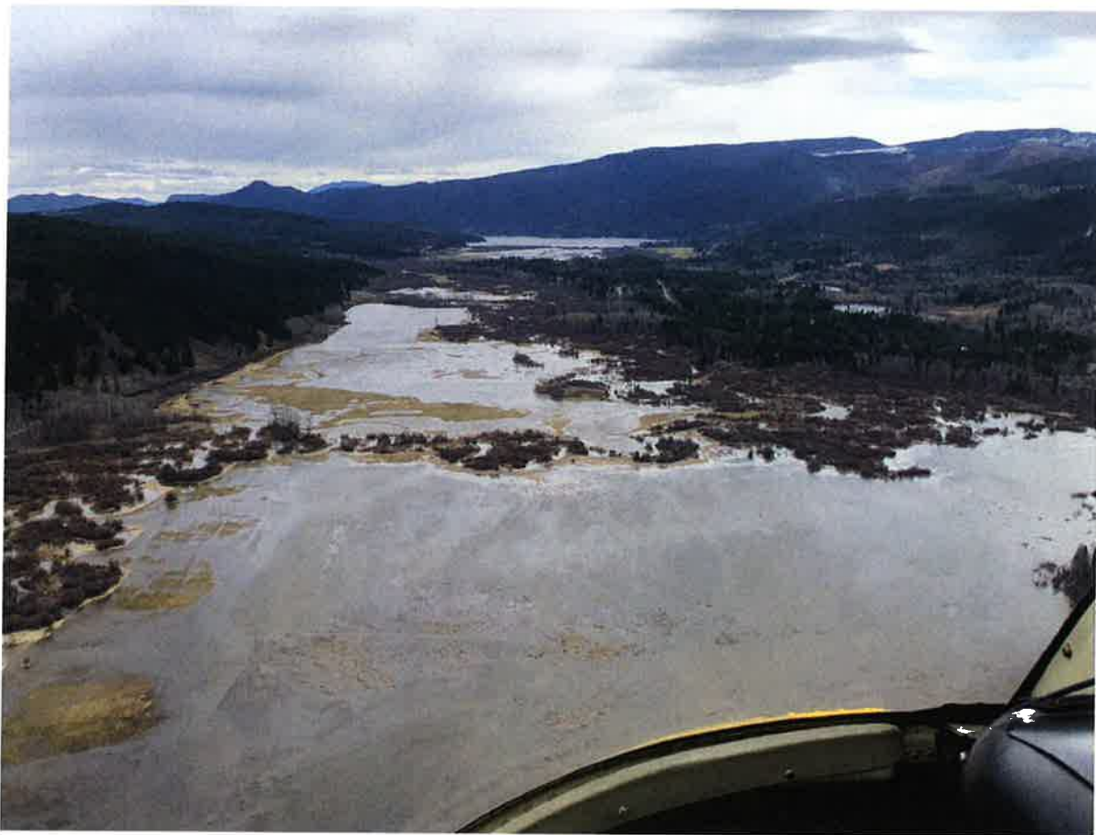
Figure 1-3. View east across flooded areas of Bridge Creek near Canim Lake, Tso'escen Road in foreground (Canim Lake Band Reserve) (May 2, 2020, Photo Courtesy CRD, 2020).
