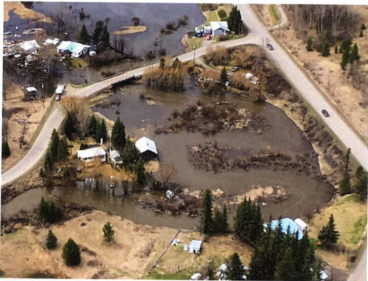
Figure 1-1. View of flooded properties at Houseman Road, looking south at Houseman Bridge within the CRD. (May 2, 2020, Photo Courtesy CRD, 2020).
