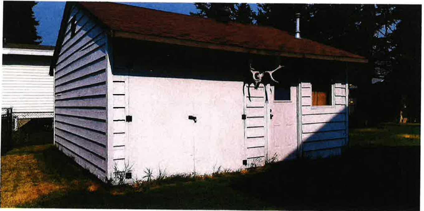
Workshop 182 Evergreen Crescent
