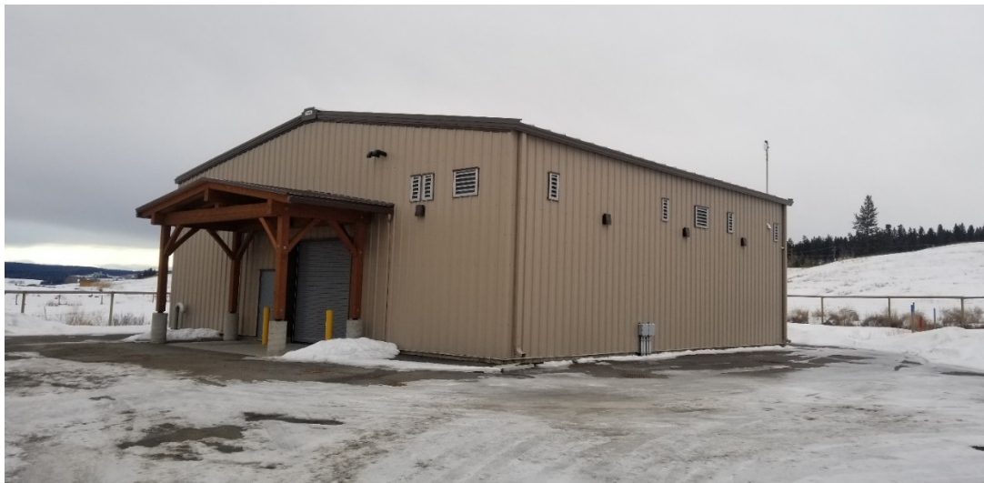
Figure 1: The District of 100 Mile House Water Treatment Plant
