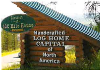
CURRENT LETTERS WILL NEED TO BE REMOVED; LOGS TO BE SANDED AND REFINISHED LIGHTLY BEFORE INSTALLATION.
