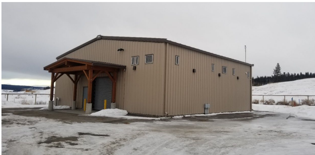
Figure 1: The District of 100 Mile House Water Treatment Plan
